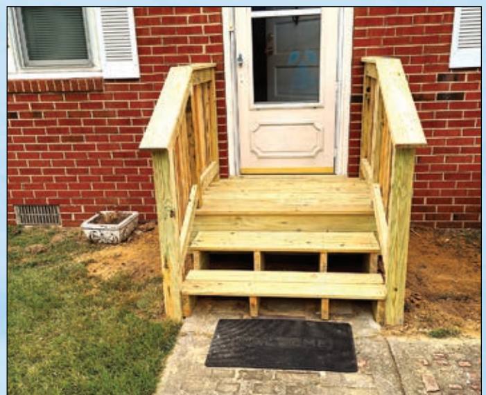
Entrance stairs repaired for senior Tribal members.
