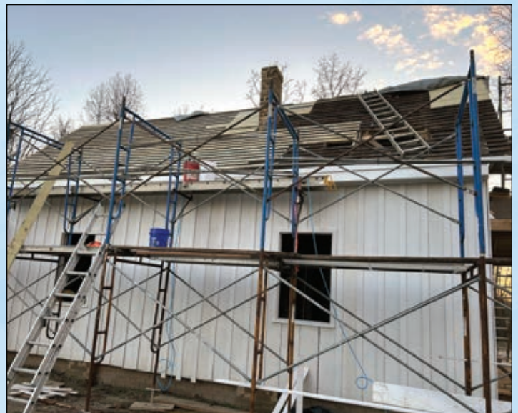
Chiefs House project work progress in October, 2023.
