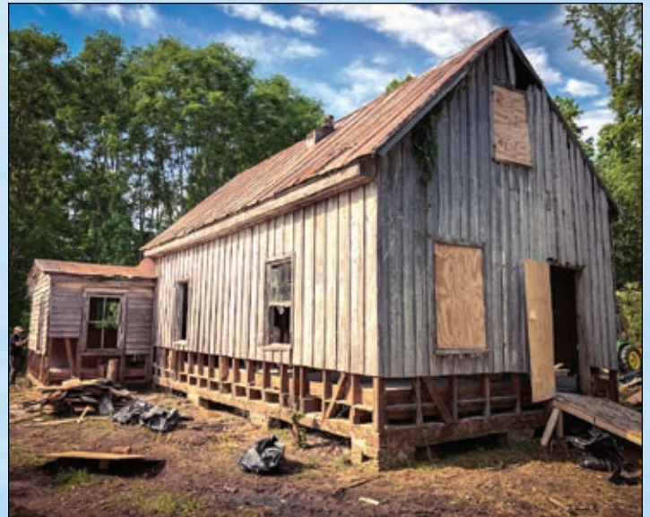
Chiefs House project work progress in June, 2023.
