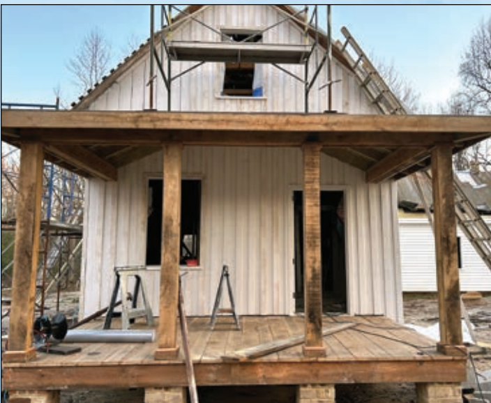
Chiefs House project work progress in October, 2023.
