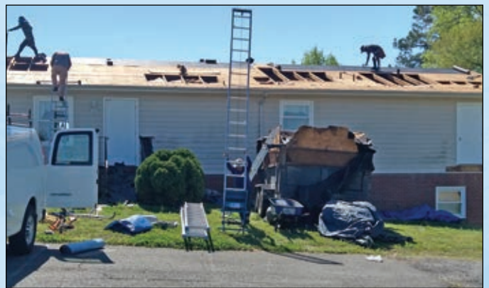
New roof installation at the dental clinic building.
