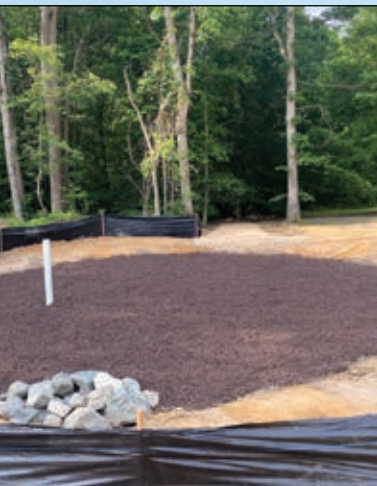
Bioretention structure at the Tribal Center to prevent flooding, under construction on left, completed on right.
