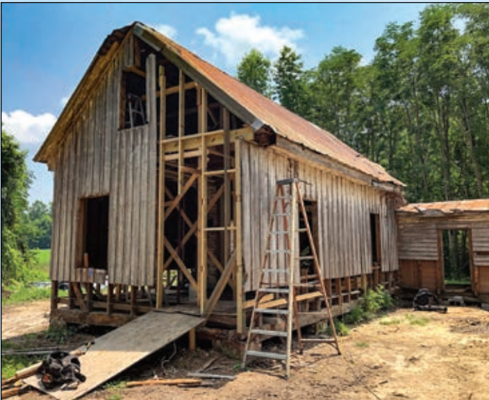
Chiefs House project work progress in April, 2023.
