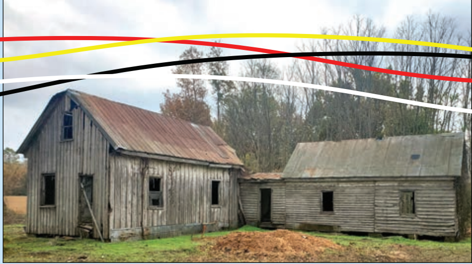
Chiefs house before rehabilitation project work began.
