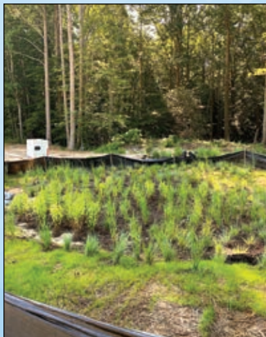
Bioretention structure at the Tribal Center to prevent flooding, under construction on left, completed on right.
