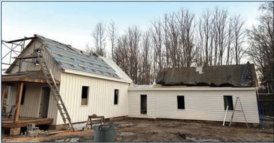
Chiefs House project work progress in October, 2023.
