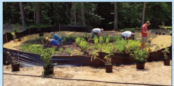
Creating a new drainage retention area.
