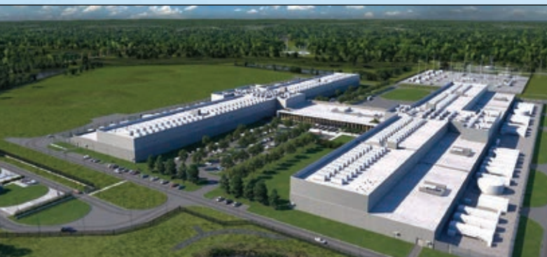
Planned data center in Central Virginia Photo from Virginia Economic Development Partnership.
