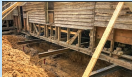
Chiefs House has a new foundation, but original brick pilings remain.
